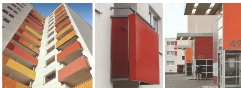
Figure 3 Strucksburg housing façade, Hamburg, Germany [9]
