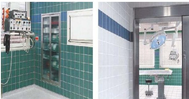
Figure 7 Operating theatre, Goslar, Germany [16]
