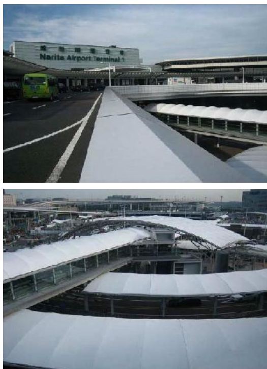
Figure 4 Narita International Airport of Tokyo, Terminal 1, Chiba, Japan [14]
