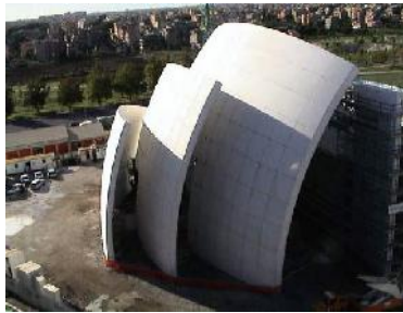
Figure 14 Construction of the Church (sails) [20]
