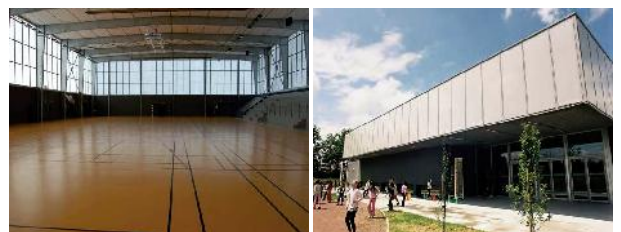
Figure 11 Sports hall, Carquefou, ZAC du Souchais, France (internal and external view) [18]
