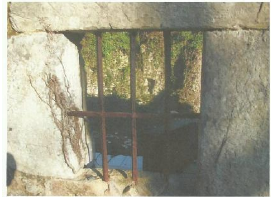
Figure.4 Image showing the state of the iron bars taken is observed to take samples of the mill Zabale-Errota.
