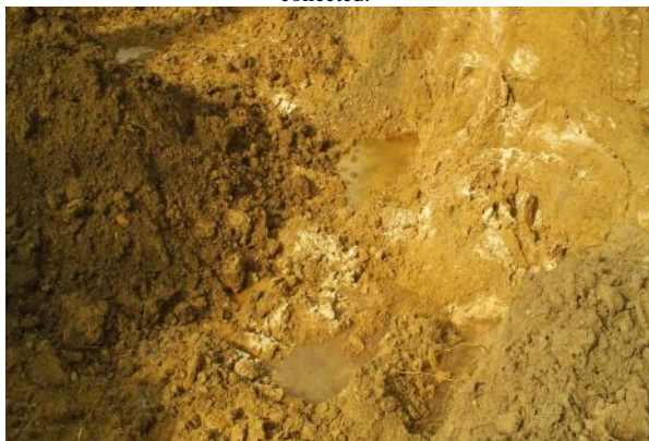
Figure 14 Showing backfilling of excavated soil, after direct application of bionutrient on the surface of the exposed underground water.
